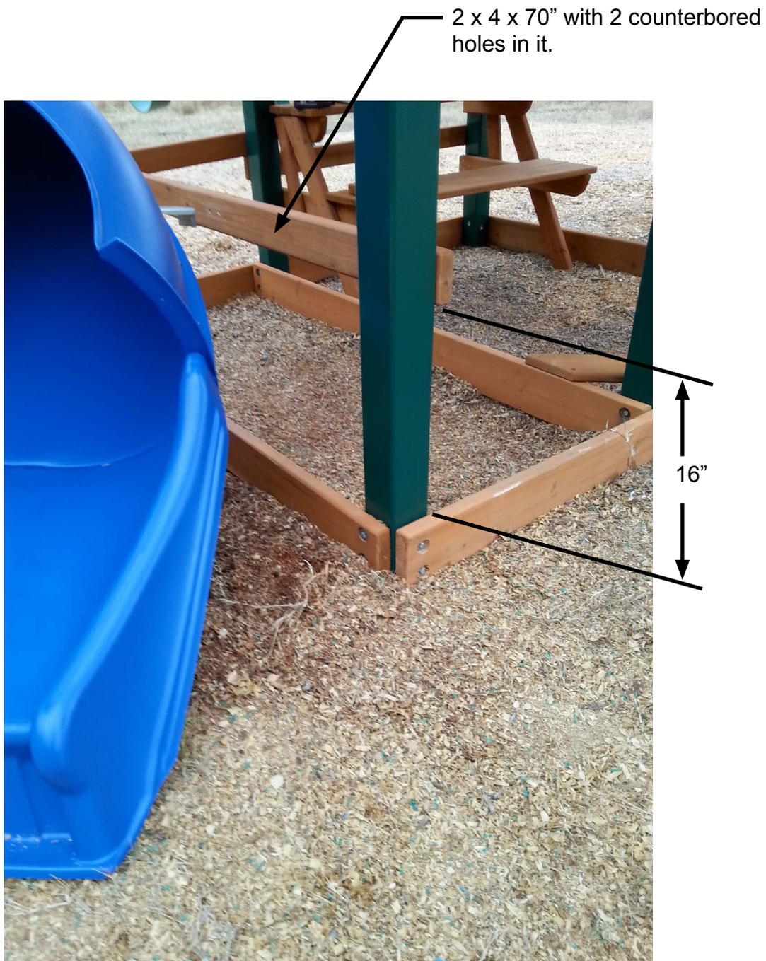
1. Place the 5/16" x 2-3/4" hex bolts with washers through the holes in the slide bracket and then through the holes in the 2 x 4 x 4" long board with 2 holes in it. Align the top of the 4" board to the top of the 2 x 4 x 70" board as best as you are able. Then use a hammer to strike the end of each bolt to leave a mark on the 2 x 4 x 70" board.
